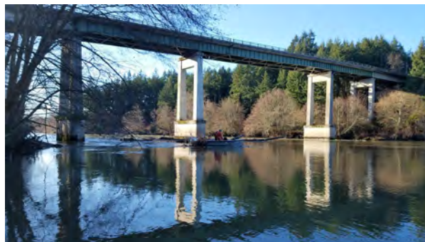
North Fork Bridge Debris Removal 2017
