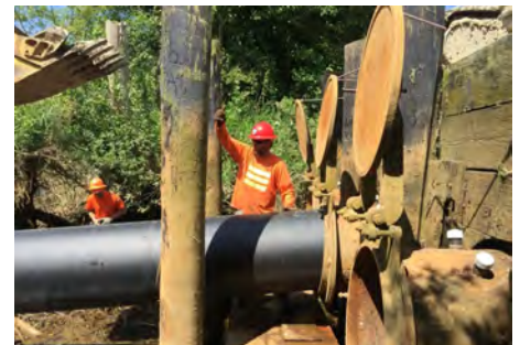
Chilberg Pump Discharge Pipe Lining
