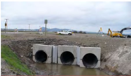
No Name Slough Bypass Culverts
