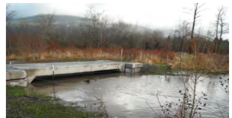
Red Creek Culvert Replacement
