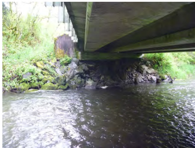
Friday Creek Bridge 2017 Inspection
