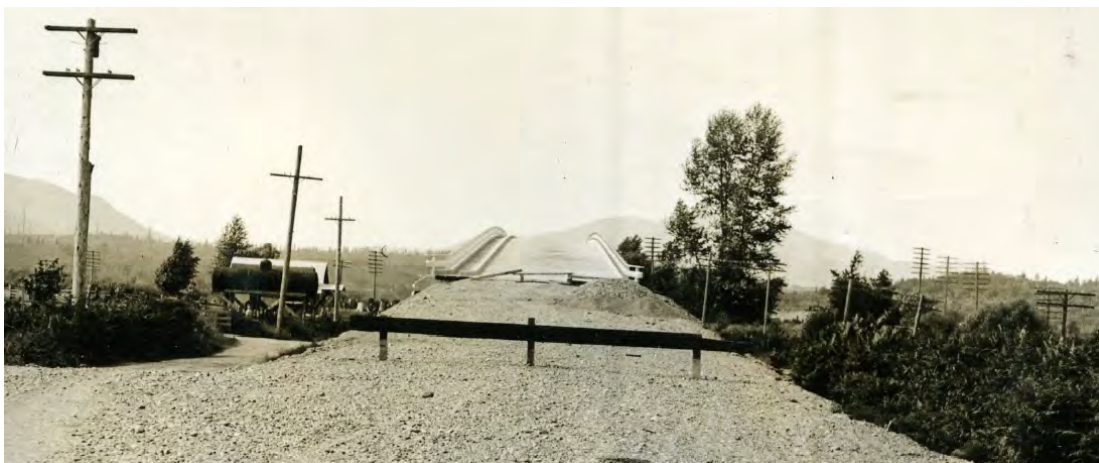
1936 Burlington Northern Overpass Construction
