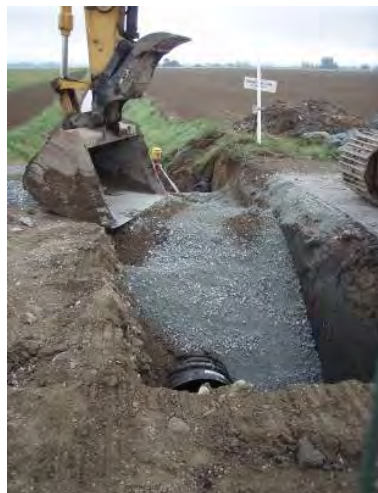
Maupin Road Conveyance Improvement Dike & Drainage District 22 (2008)
