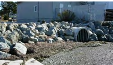
Bay View Padilla Bay Culvert Extension
