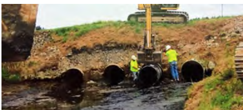
Samish Flood Return Pipe Lining
