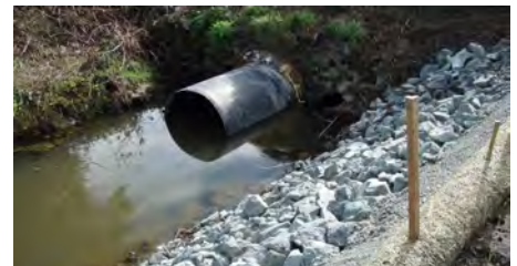
Brown Slough Pipe Lining
